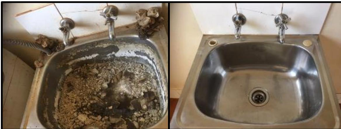
Figure 34: Before and after pictures of blocked sink. Courtesy of Nirrumbuk Healthy Housing hardware.
